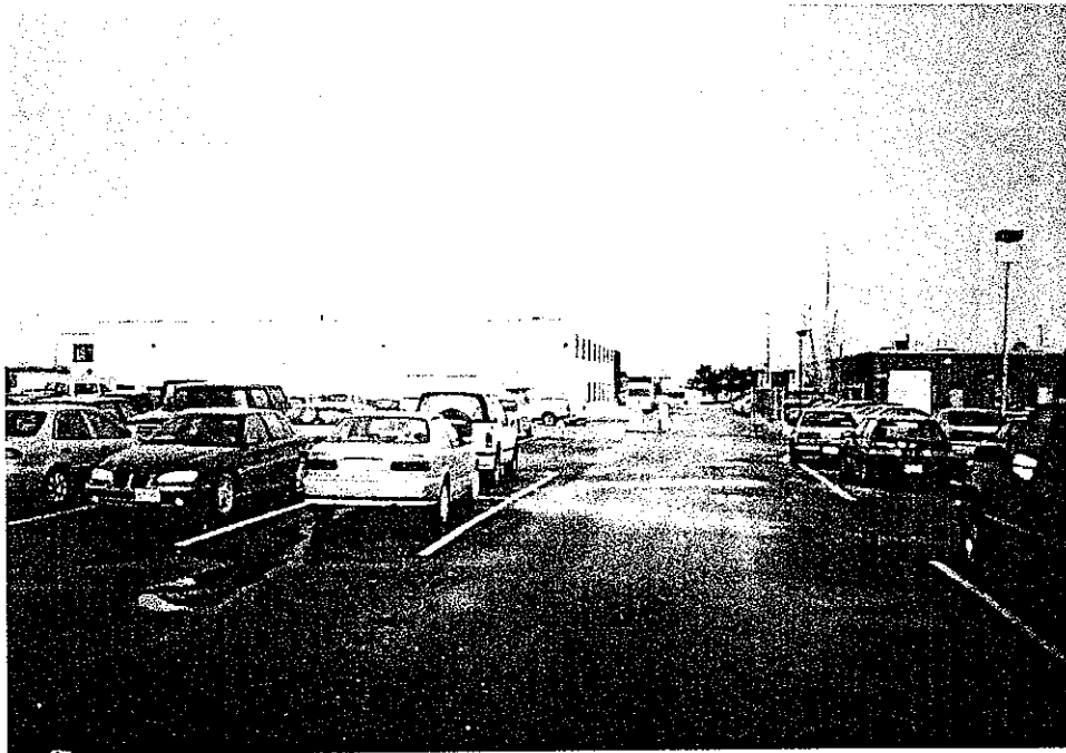
Looking north along east side of property from the parking lot towards the warehouse portion of the building.
