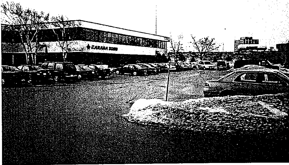
View of north side of building looking southwest. Truck in background is on Highway 427 overpass.
